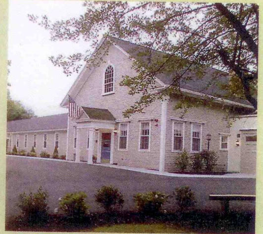
LARGE CATEGORY WINNER: LEXINGTON - DOUGLAS HOUSE Lexington's Douglas House provides 15 affordable housing units for survivors of serious brain injuries. This project meets three CPA purposes: historic preservation, affordable housing and recreation. The proximity of Lexington's downtown area, its public transportation, its cultural amenities and the prospect of local jobs made this former home of the Lexington Press an ideal location for this project.
